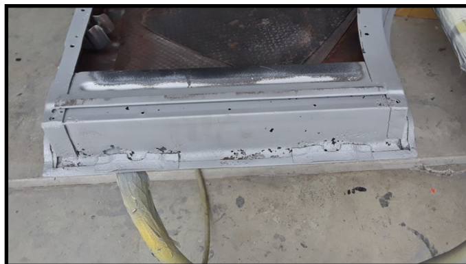
Rust in the cowl, driver's side
